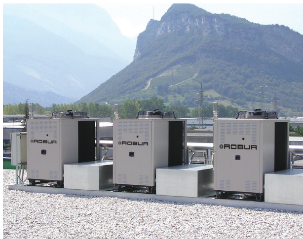
Fig.1 - Installation of reversible absorption heat pumps on the building roof.
